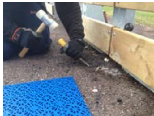
Example of laying/smoothing
